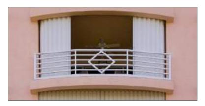
The accordion shutters' ability to cover wide spans, such as lanais and balconies, as well as ease of use, make Roll-a-way Accordion Shutters one of our most popular storm protection solutions.
