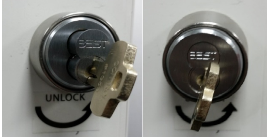
Picture 7: Left is halfway inserted; Right is fully inserted flush
